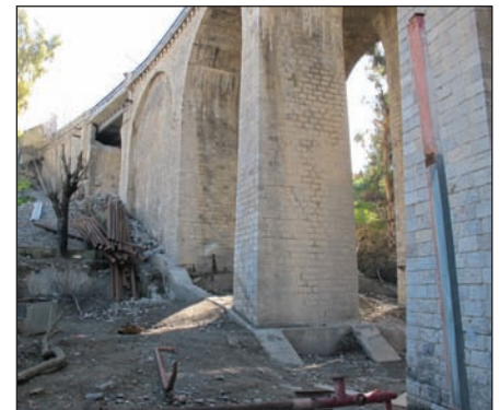
Fig. 3: Existing reinforced concrete beams connecting the foundations of the piers
