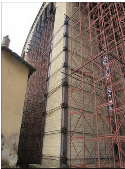
Fig. 7: Emergency propping and pier jacking with steel profiles and external posttensioning
