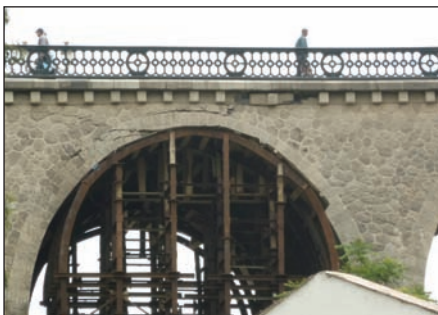
Fig. 4: Crushing of the arch between Pier 4 and 5
