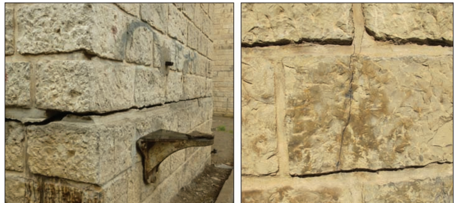
Fig. 6: Cracks at the pier bases caused by the section rotation: (left) mode-I opening on the tensile side; (right) splitting cracks on the compression zone
