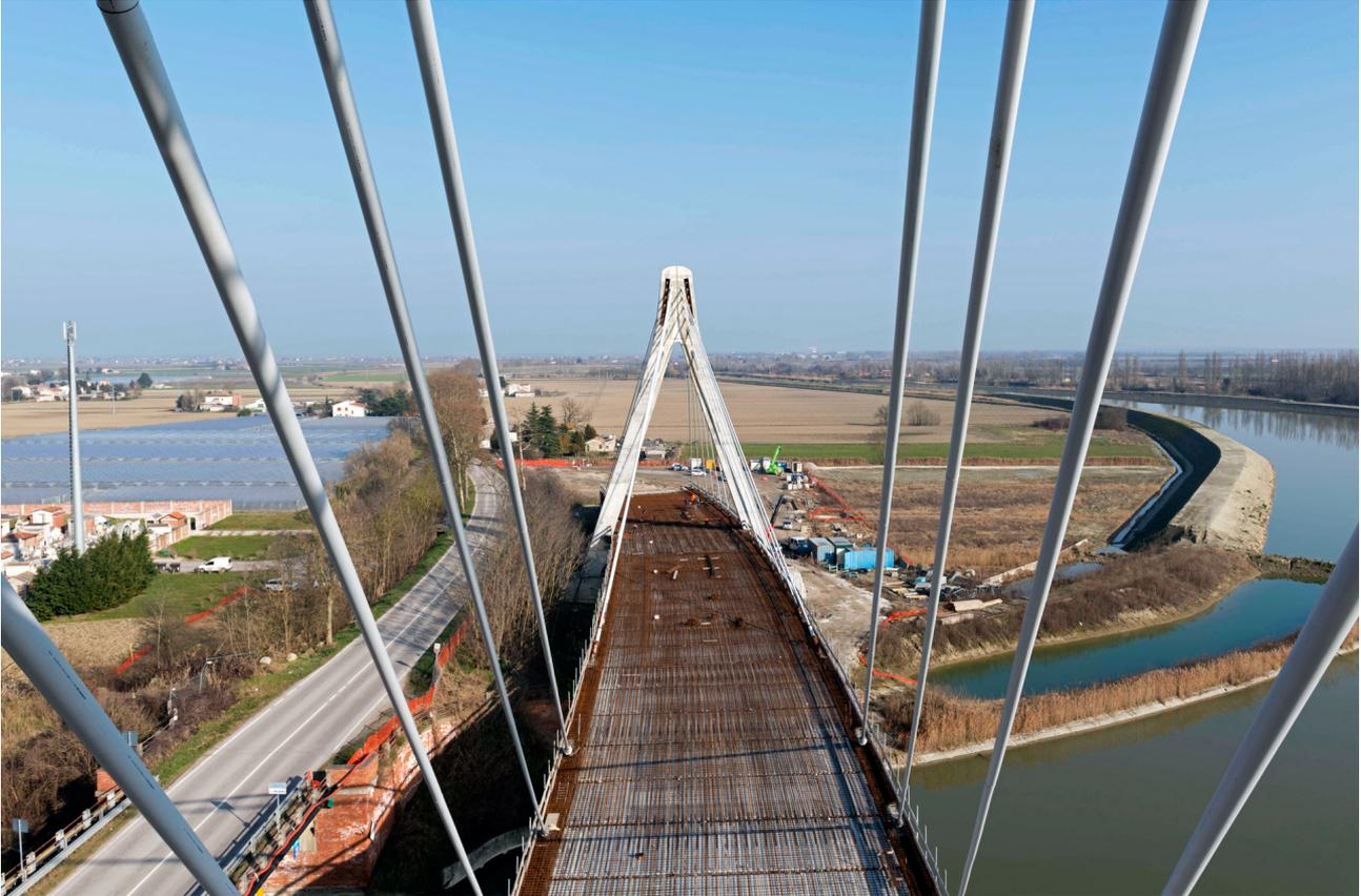
*Fig. 7: The deck slab under construction*
