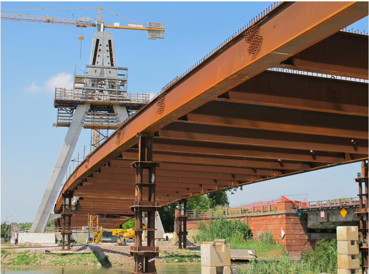
*Fig. 5: The steel deck*
